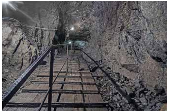
The unexpected ramp that links two levels in the Osowka complex. Some believe this was necessary to overcome geological faulting. Photo Chris Wilkins
